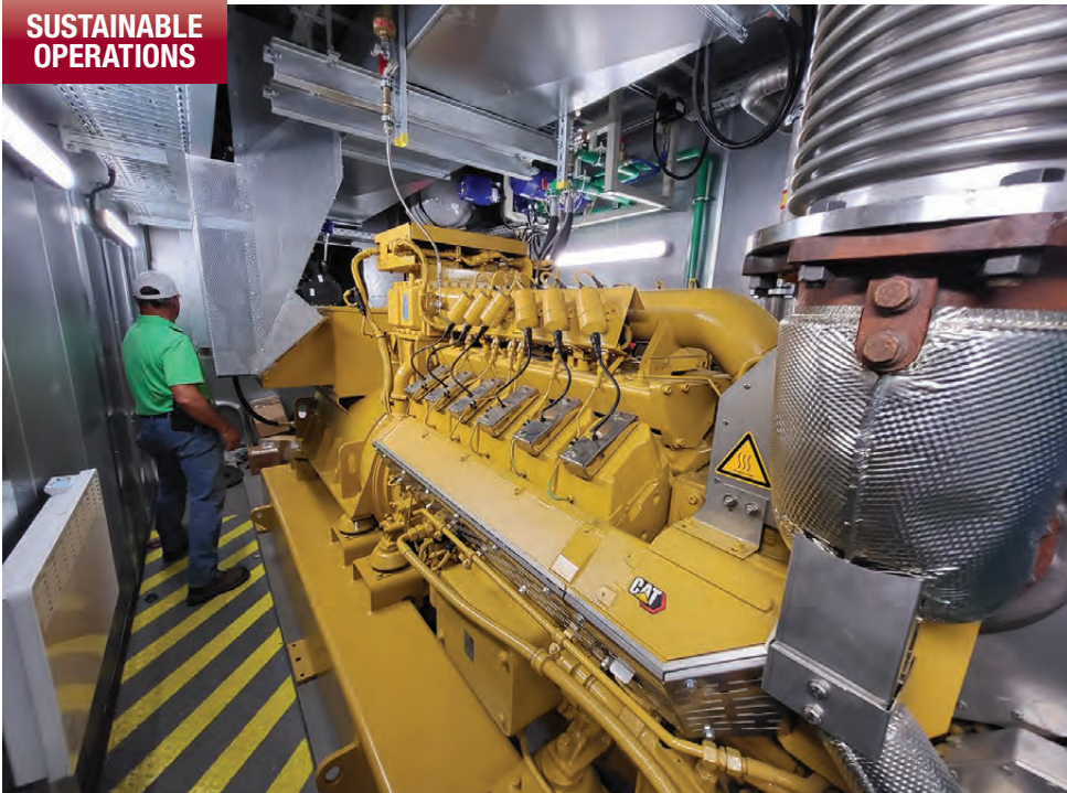
ABOVE: The project has paid dividends that include avoidance of high compliance costs, cleaner operation and resiliency, both locally and regionally. LEFT: The combined heat and power system includes two biogas-fueled 600 kW Caterpillar engine-generators that together can supply up to 80% of the treatment plant's demand.
